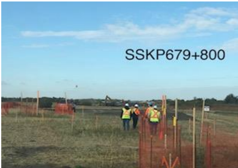
Access ramp installation near organic field
