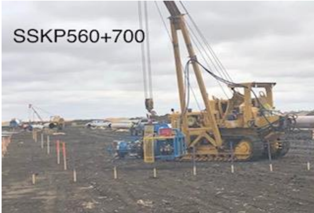
Bevelling crew prepping for welding
