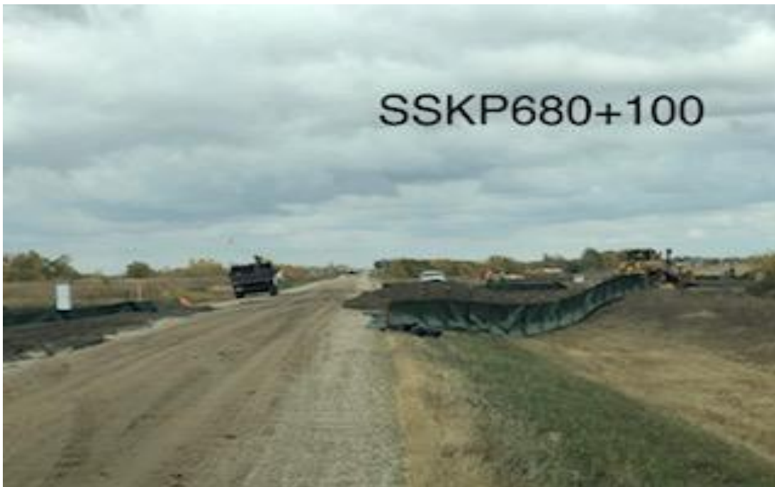
Access ramp Geotech and wingwall installation
