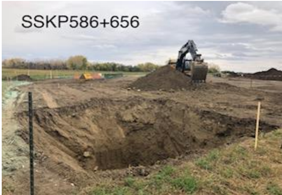
Cradle Bore excavation
