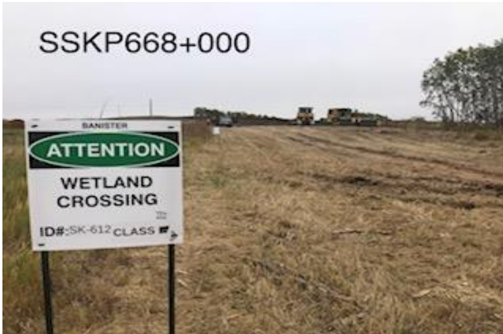
Power Dozer Near Wet Land Crossing
