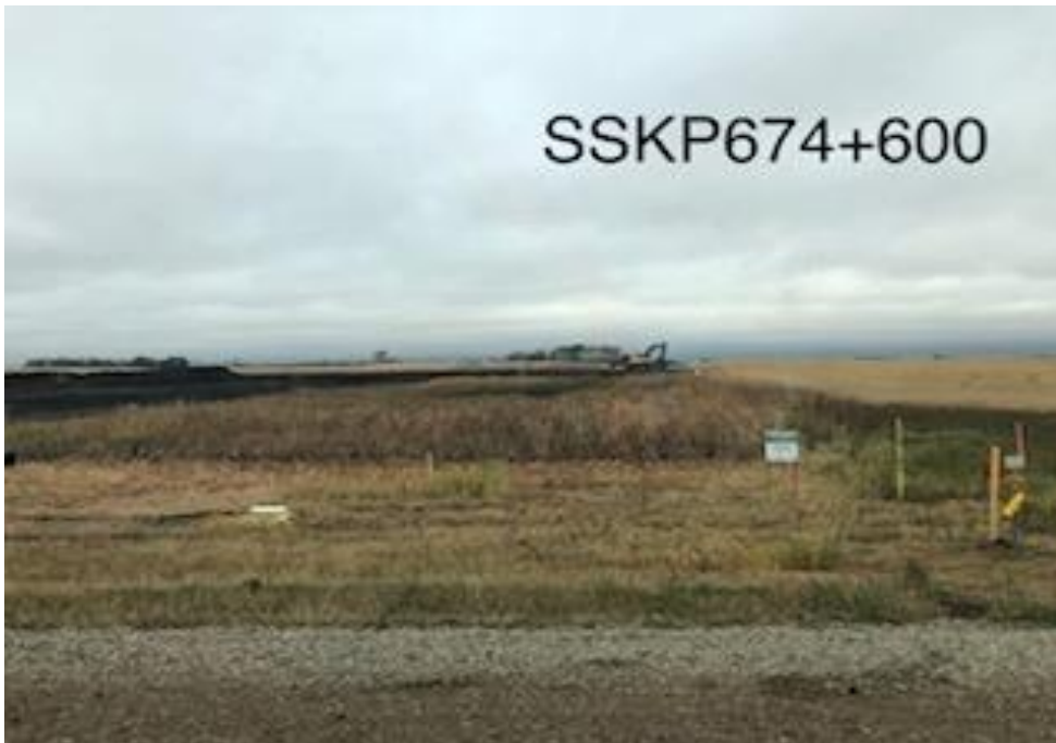
Access and Grade near Wet Land
